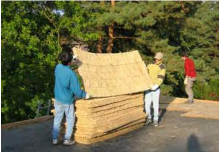
Reed insulation on green roof. Photo by Achim Ecker.
