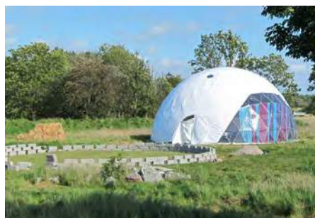
Dome shaped building as a greenhouse at Suderbyn Ecovillage, Sweden. Photo by Mia Saloranta.
