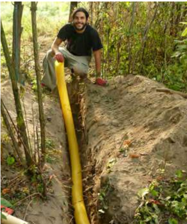
Building a natural waste water purification system. Photo by Monika Podsiadła.
