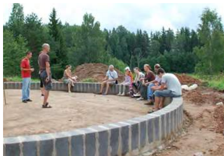
Foundation for dome house in Jaunpiebalga. Photo by Daina Saktiņa.
