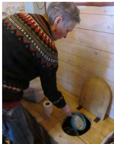
Sawdust is added to the compost toilet after use. In the photo you can see the urine separating unit in the toilet hole, adapted from a plastic funnel. Photo by Mia Saloranta.
