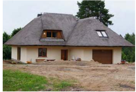
Straw bale house at Domantas Surkys ecovillage. Photo by Živilė Gedminaitė-Raudonė.
