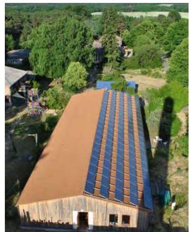
Finished solar thermal roof from above. Photo by Achim Ecker.
