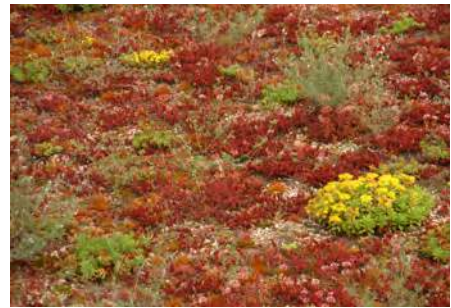
Green insulated roof. Photo by Achim Ecker.
