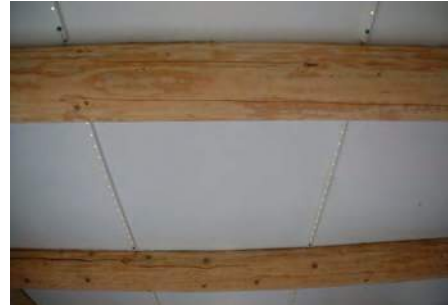
Room lighting system in family house. Photo by Daina Saktiņa.
