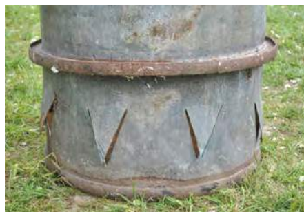
Detail of openings for air inflow, at the bottom of the big oil barrel. Photo by Jesús Pacheco Justo.
