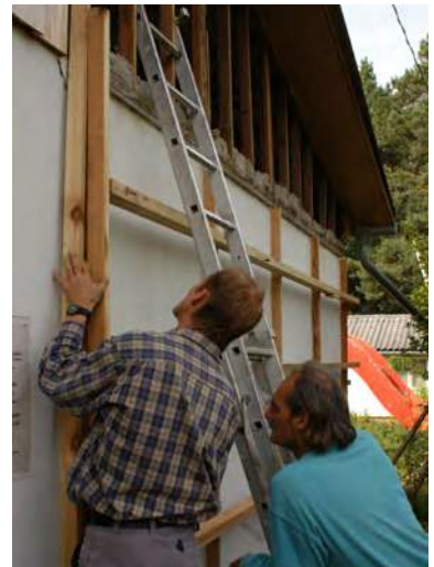
Insulation (foam glass and cellulose fibres). Photo by Achim Ecker.
