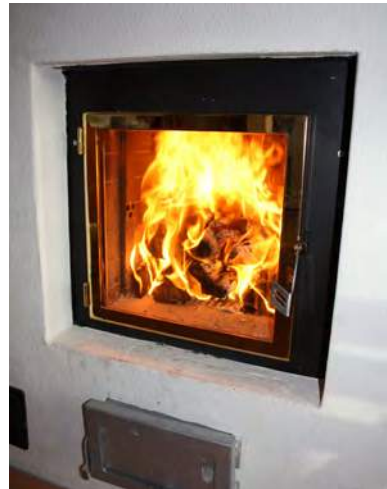
The vents that direct secondary air to the flames. Photo by Ella Suhonen.
