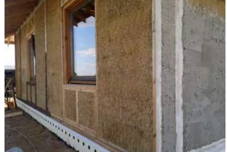
Plastering the walls of a straw house. Photo by Domantas Surkys.
