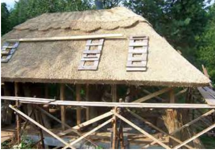
Building a straw house. Photo by Domantas Surkys.
