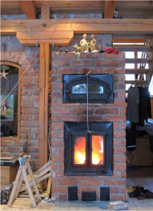
Fireplace made of recycled bricks. Photo by Mia Saloranta.
