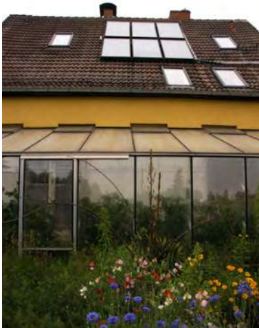
Solar thermal panels of a separate house with greenhouse near our organic garden. Photo by Achim Ecker.
