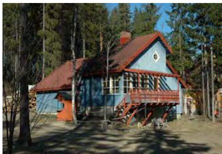
The heating plant with recycled windows. Behind the building you can see a pile of wood waiting to be chipped. Photo by Outi Palttala.
